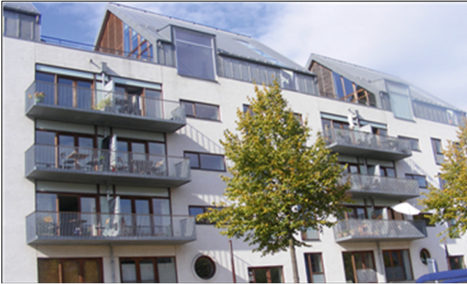
Fig. 3. Rooftop extension (SOLTAG system) in the City Copenhagen, Denmark [6]
